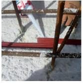
4. Make the overlap by placing the joint parallel to each other for about 5 cm. Do not overlap. We can use MS Polymer to regularize the support Art. No. 1893100191 - 310ml or Art. No. 0892320020 - 600ml.
